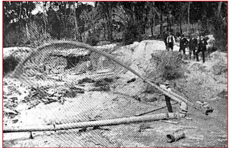
Near view of Nozzle showing how the direction of water is controlled
