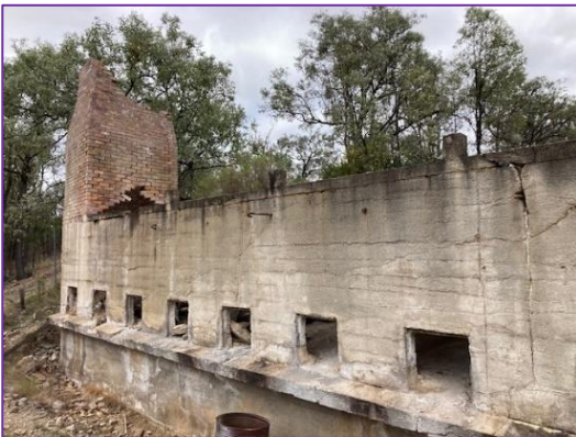
Arsenic pentoxide cooling chambers
